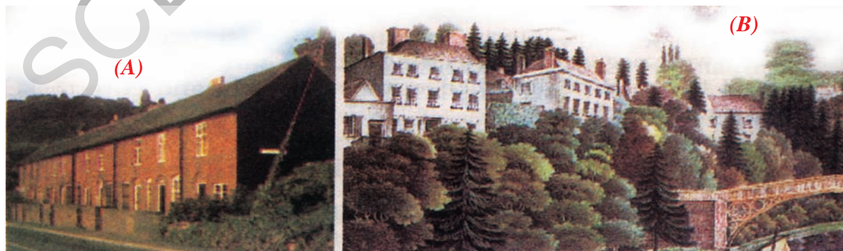
Fig. 13.4: (A) Coalbrookdale, Carpenters' Row, cottages built by the company for workers in 1783 CE; (B) The houses of the Darbys; painting by William Westwood, 1835 CE.
