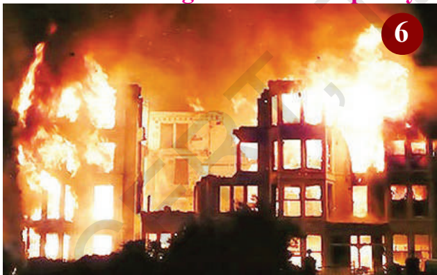
Fire accidents in an apartment
