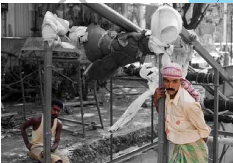
Fig 19.5 Road Laying Work
