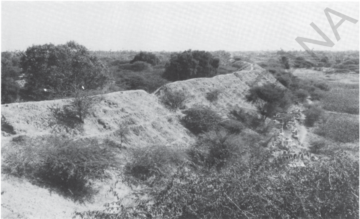
Fig 12.3 A segment of the inner earthen wall with its (dry) moat at right
