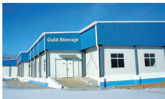
Fig-28 : Cold storage unit
