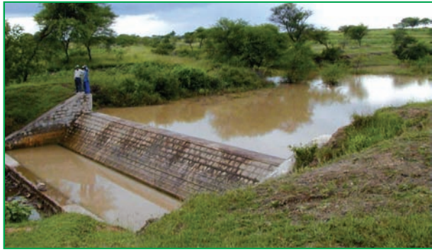
Fig-1: Community based masonry dam
