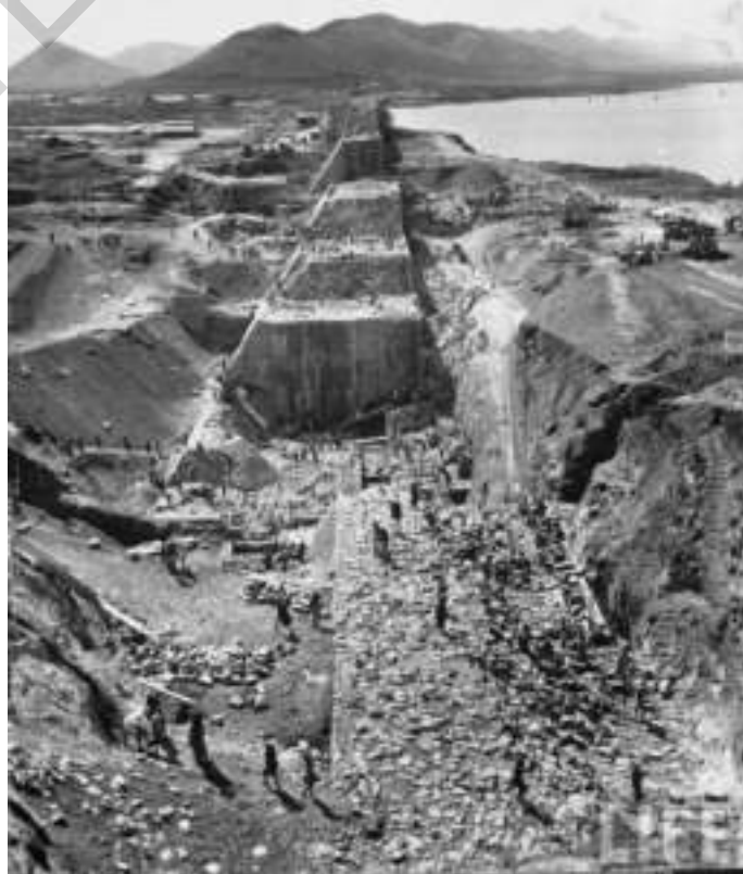
Fig 5.1 : Tungabhadra Dam Construction - 1952
